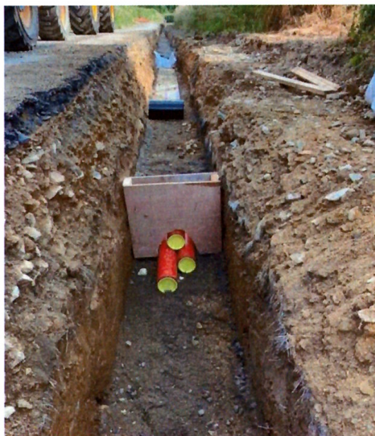
Figure 5-4 Typical 33KV Underground Duct Installation
